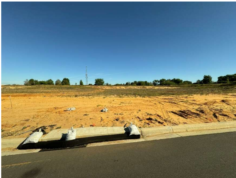
Windsor Cay CDD West side of U.S. Highway 27, south of County Road 474 Clermont, Florida
